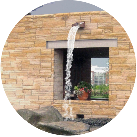
Wall scupper: water discharges from stormwater detention/retention chamber under parking through scupper in retaining wall to raingarden below
